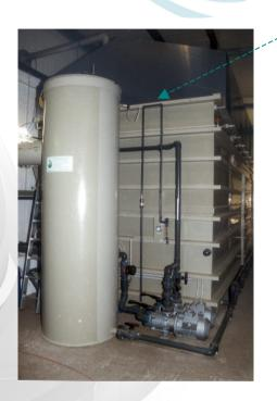
Gas supply line guidance above highest liquid-level in order to avoid that water will attain the air flow measuring device (3)
