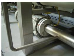
Design inflow pipe for the range of air inlet til pump inlet flange in a short and horizontal way in order to ensure that always a constant water-air proportion arrives at the pump
